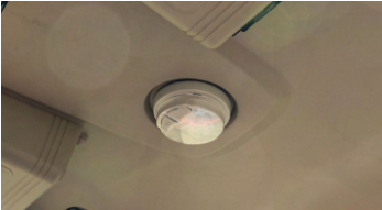
4. LED interior lighting
